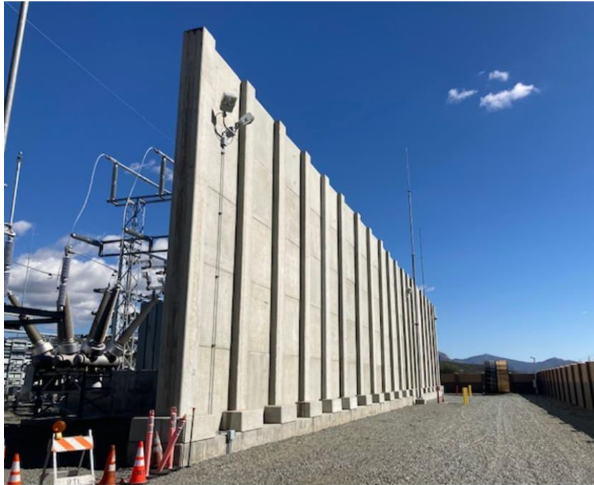
Figure HWT 8.1.2-1. Transformer Fire Barrier Wall
