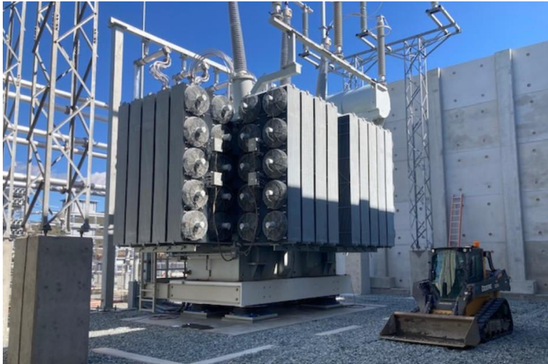
Figure HWT 8.1.2-3. Transformer Seismic Isolation Pad
